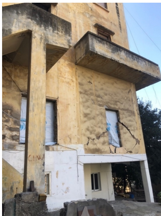
Figure 2. Structurally damaged building along Fouad Boutros trajectory. Source: Luna Dayekh, 2020
