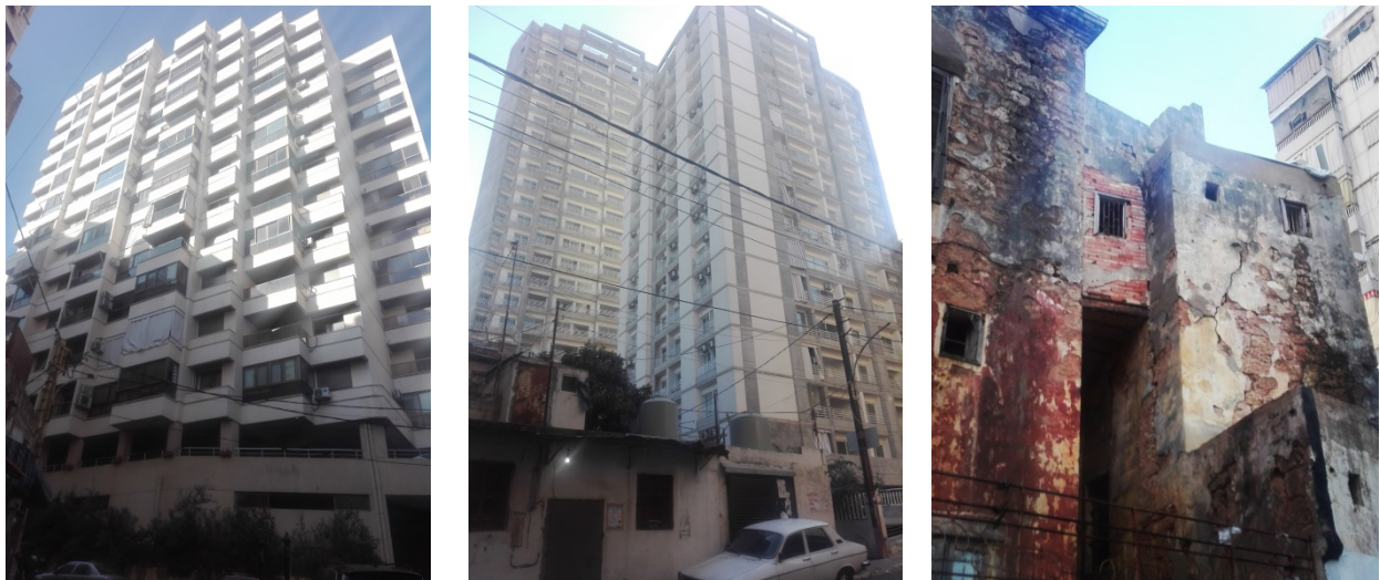
Figure 4. New development and abandoned decaying heritage buildings. Source: Lynn Hamdar and Fatima Alleik, 2020.
