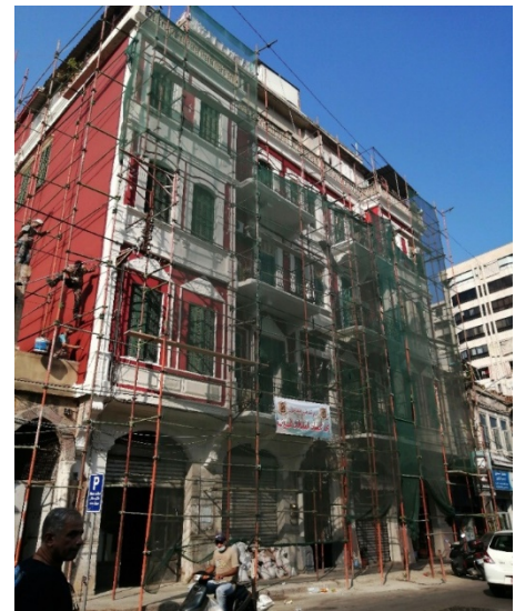
Figure 21. Old Building being renovated by the League of Beiruti Families after the port's blast. Source: Lynn Hamdar and Fatima Alleik, 2020.
