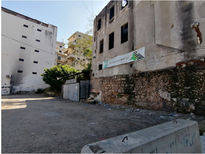
Figure 16. Street-level generator located at the edge of BDD zone. Source: Lynn Hamdar and Fatima Alleik, 2020.
