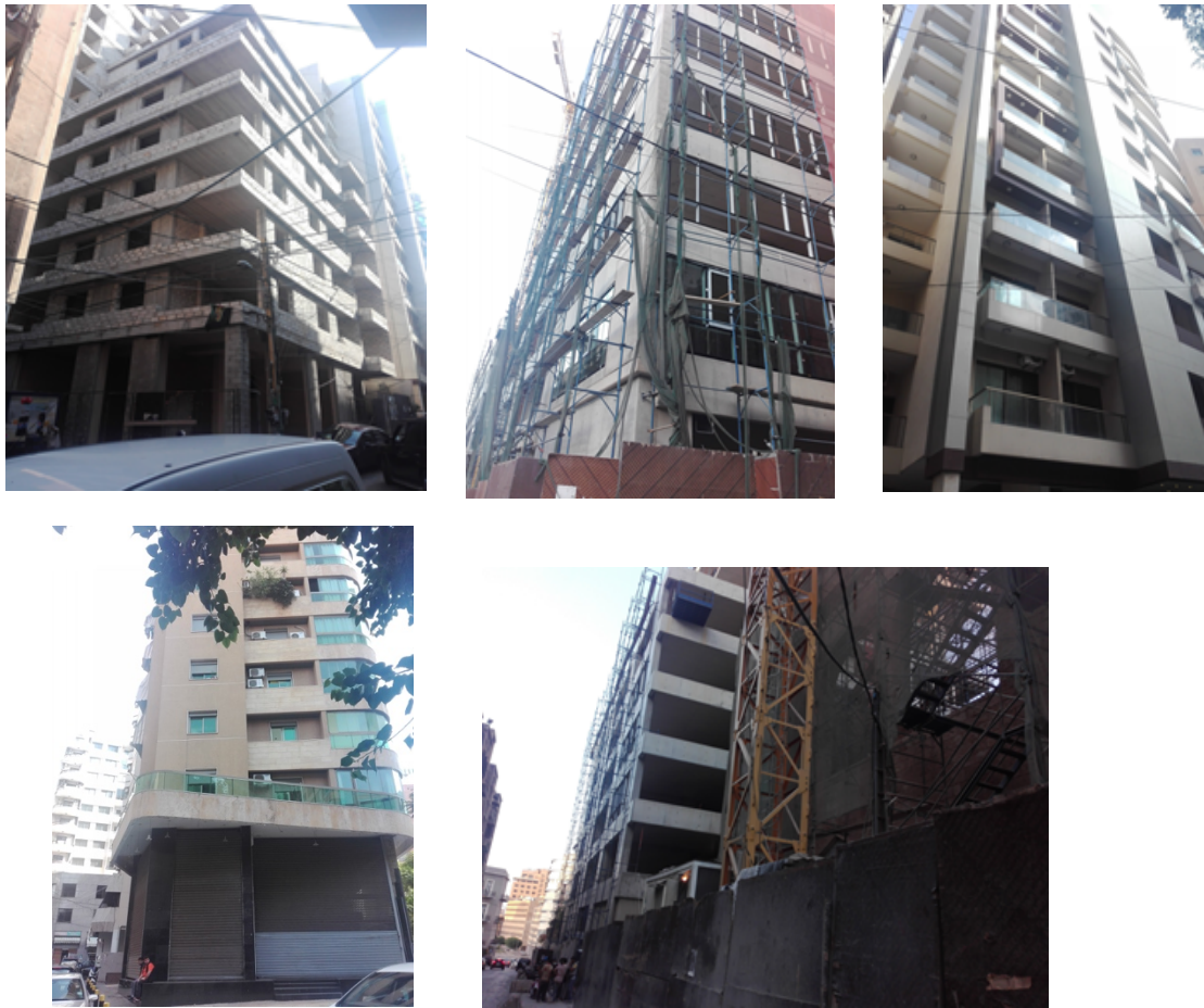
Figure 3. New construction in BDD (bottom) and residential towers (top) along Ibrahim el-Ahdab Street. Source: Lynn Hamdar and Fatima Alleik, 2020.
