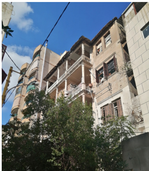
Figure 8. Partially Abandoned Building in Basta al-Tahta. Source: Lynn Hamdar and Fatima Alleik, 2020.
