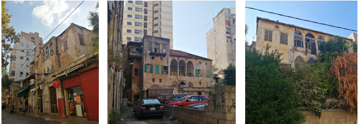
Figure 7. Heritage building in Basta al-Tahta,. Source: Lynn Hamdar and Fatima Alleik, November 16th and 30th 2020. Five housing units were later rehabilitated by UNHCR and a local NGO, in December 2020.
