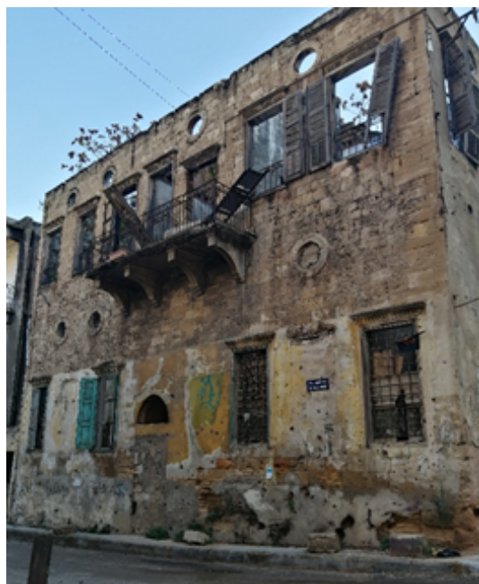
Figure 6. Abandoned heritage building in the Christian Neighborhood. Source: Lynn Hamdar and Fatima Alleik, 2020.
