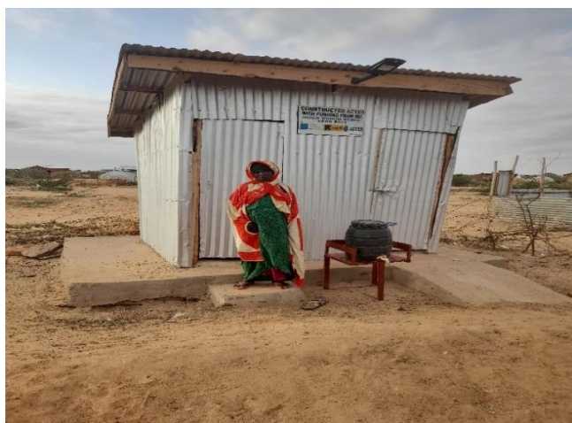
Laila in front of the double-door latrine (with solar light and handwashing facility) at Arra'ad Site, Dollo Ado Woreda, Liben Zone
