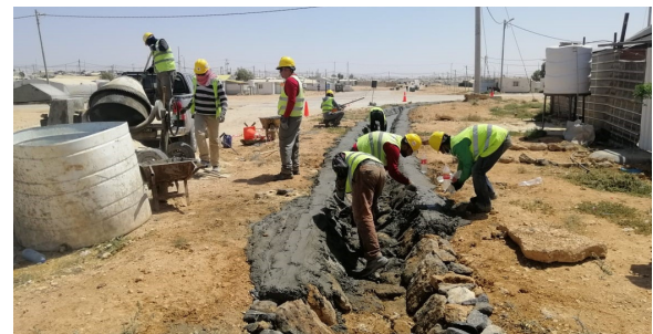
Construction of the drainage system by camp residents, September 2020
