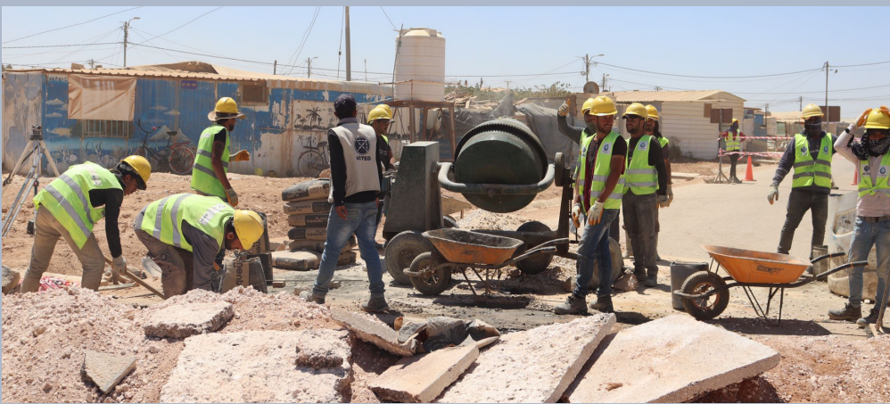
Construction works during August, 2022
