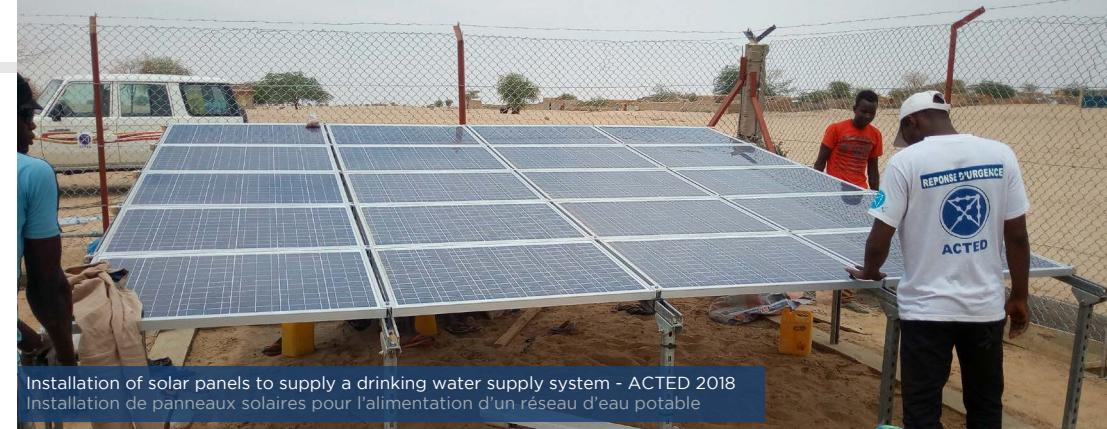
Installation of solar panels to supply a drinking water supply system - ACTED 2018
