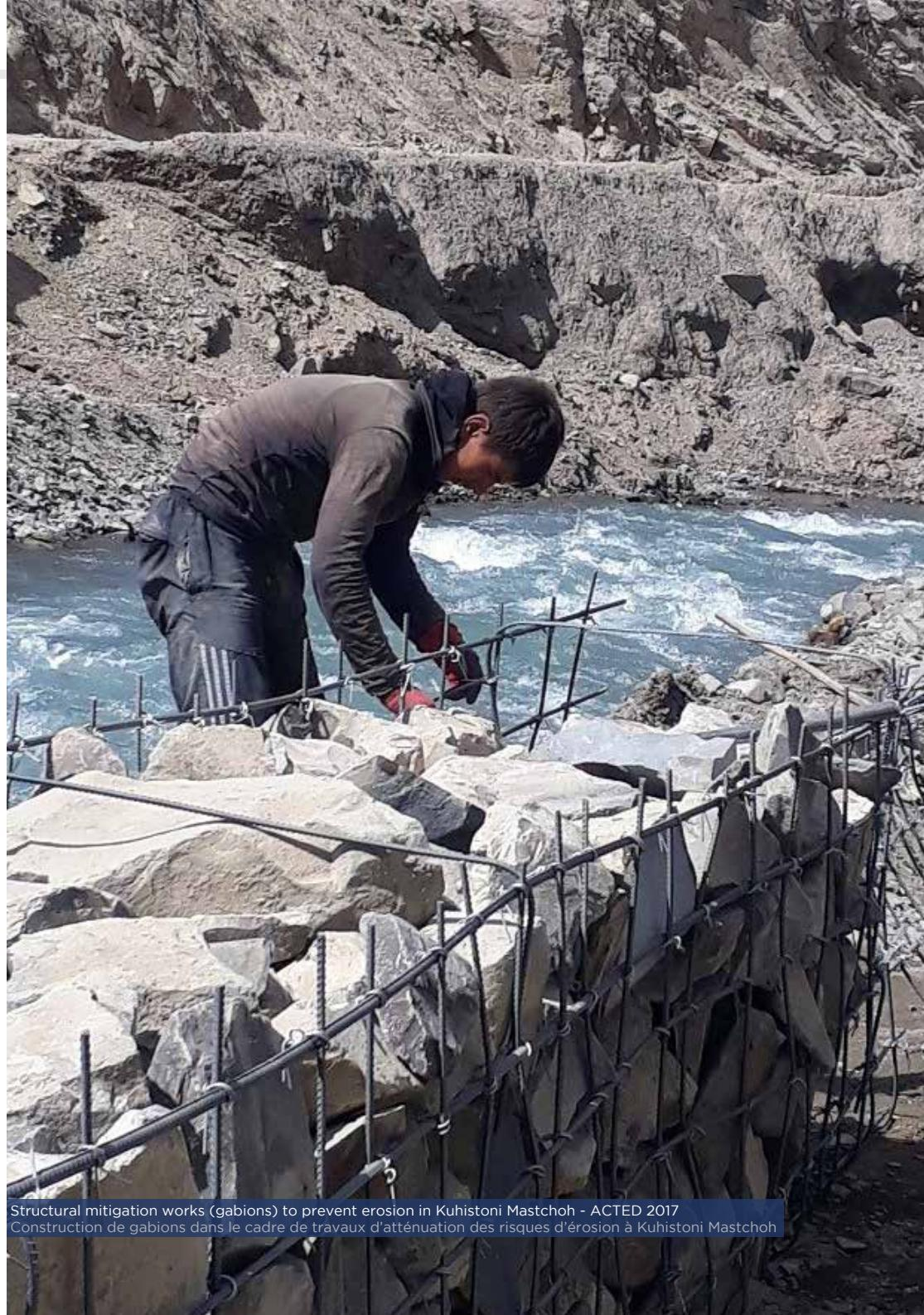
Structural mitigation works (gabions) to prevent erosion in Kuhistoni Mastchoh - ACTED 2017
