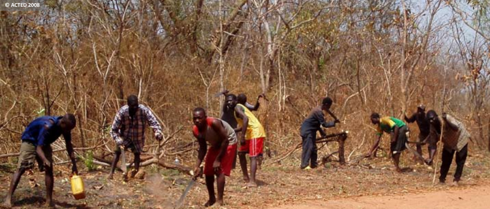
Digging of gutters - rehabilitation of the Kaga Bandoro - Oaundago axis
