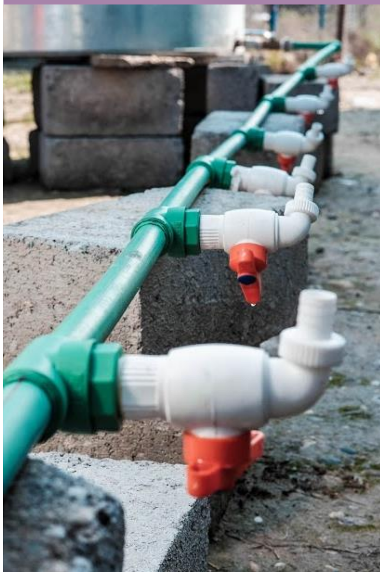
Unreliable water supply
