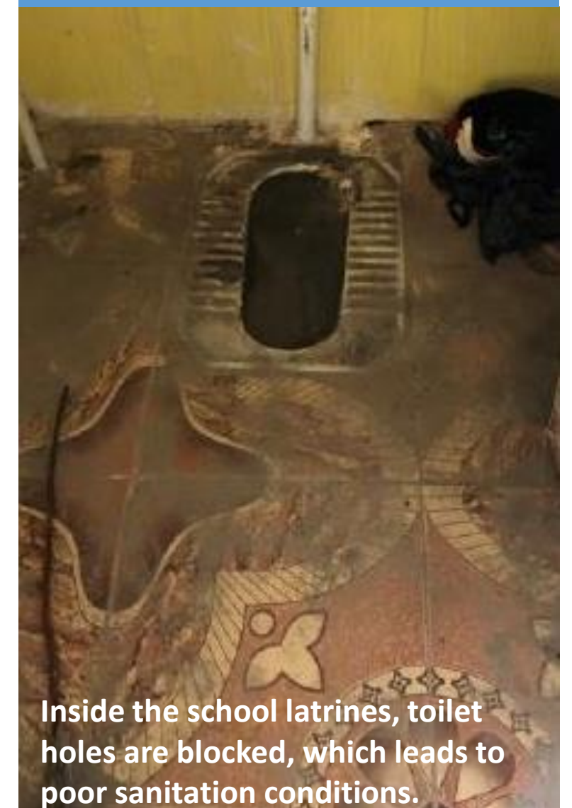
Partially functional latrines
